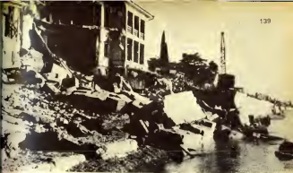
Disastrous consequences of an engineering mistake. Piers built in the wrong place prevented the flow of pebbles to this part of the shore. As a result the beach narrowed and the sea got to nearby buildings.
